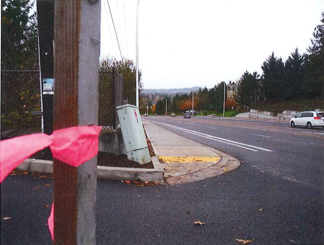
From 15 feet behind edge of traveled way of SW Scholls Ferry Rd on SW 155 th Terrace, intersection sight distance exceeds 400 feet looking east (Scholls Ferry Road)
