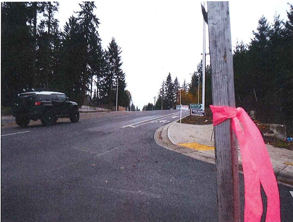
From 15 feet behind edge of traveled way of SW Scholls Ferry Rd on SW 155 th Terrace, intersection sight distance exceeds 400 feet looking west (Scholls Ferry Road)
