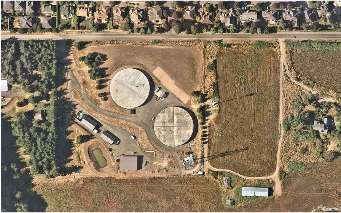
An existing water reservoir on SW Kemmer Road
