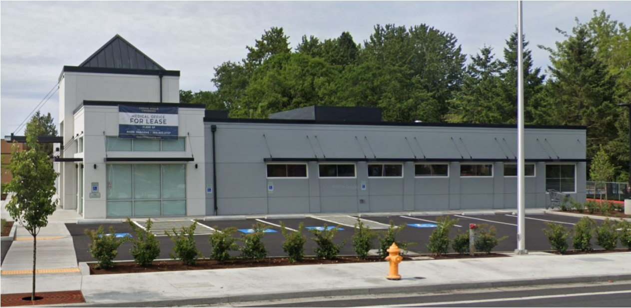
Photo 1: North Face (Facing SW Jenkins Road)
